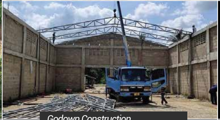
Godown Construction Dakawa - Morogoro
